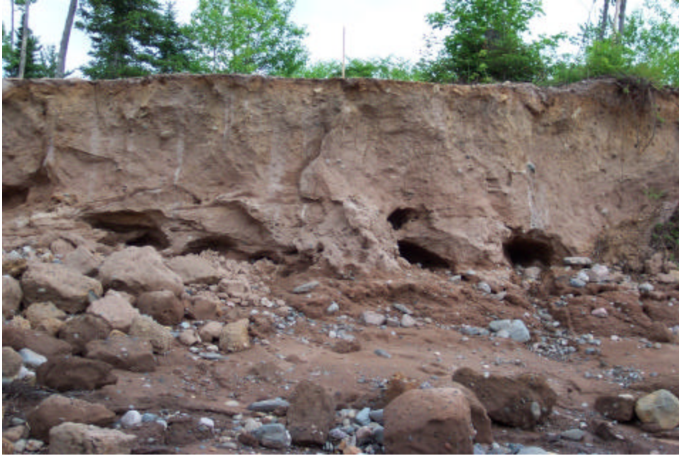
Figure 5 Note the dark brown unit immediately below the circular erosional features. This unit is a fine to medium clean sand (SP), is moist to wet, and contains prominent thin bedding (locally cross-bedded). The circular erosion appears to concentrate immediately above this change in lithology, and may be related to solution of the silt and/or carbonate content of the “coarse-textured glacial till”. View is of left channel downstream of former fuse plug.
