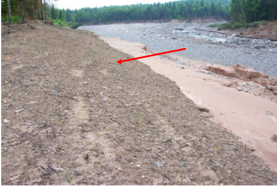
Figure 9 Foreground shows the original ground surface of the fuse plug channel. Flood erosion occurred to the right of the line marked by the arrow. Note the coarse-grained cobble and boulder deposition along the channel centerline. View is on left channel downstream of former fuse plug.
