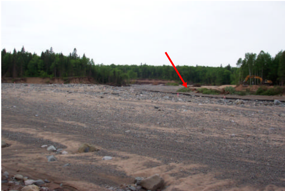
Figure 10 View of channel erosion and flood deposition downstream of former fuse plug. Note the light-colored deposits in the upper right of the photograph (arrow). This shows large amounts of well graded sand that were deposited along an inner bend of the channel alignment, approximately 1,100 feet downstream of the former fuse plug.
