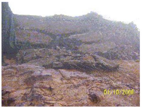
Figure 5-4. View of bedrock immediately below failed embankment section. Note weathered clay in lower portions of the exposure. (Source: FERC Staff)
