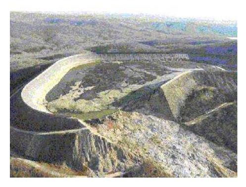
Figure 5-5. View of bedrock within, and immediately below failed embankment section. Note distribution of weathered rock (red-brown color) and topsoil (green-brown color). (Source: MDNR)
