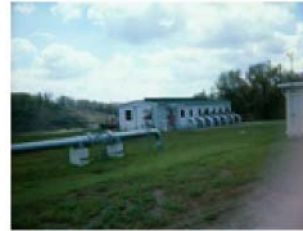
Compressor station building
