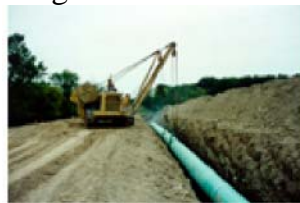
Lowering pipe in trench
