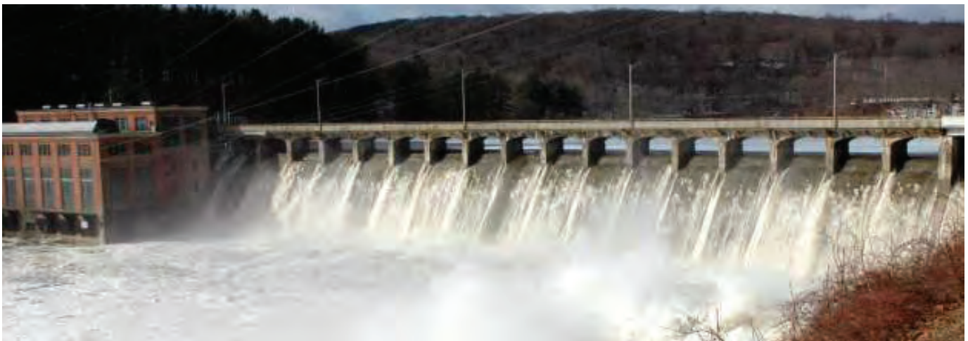
Stevenson Dam, CT
