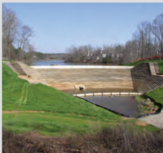
Roller Compacted Concrete
