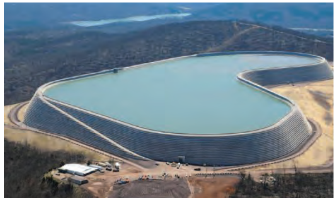
Taum Sauk rebuilt dam
