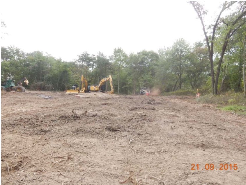
Tree clearing photograph. 9
