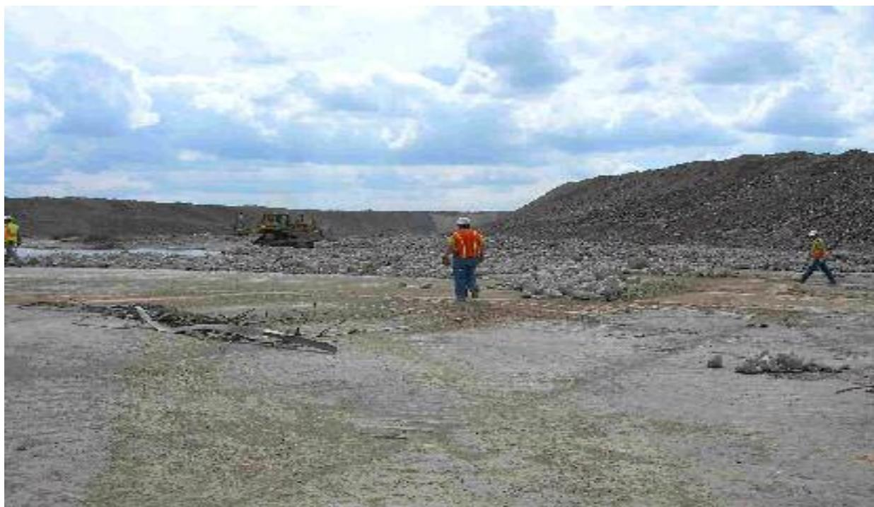
Figure 5-9. Drained upper reservoir basin showing the rockfill materials after removal of the concrete face panels. (Source: FERC Staff)
