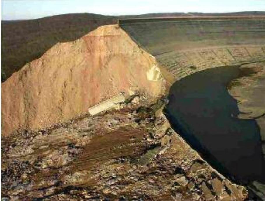
Figure 5-6. Weathered rock and discontinuous clay seam foundation just downstream of fish-pond area. (Source: FERC Staff)
