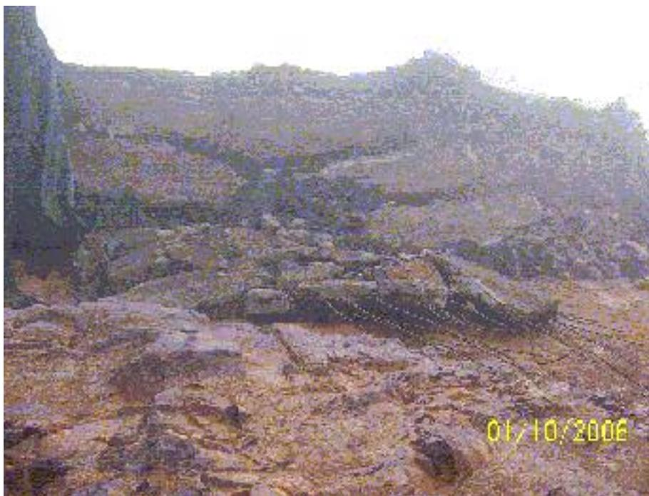
Figure 5-4. View of bedrock immediately below failed embankment section. Note weathered clay in lower portions of the exposure.
