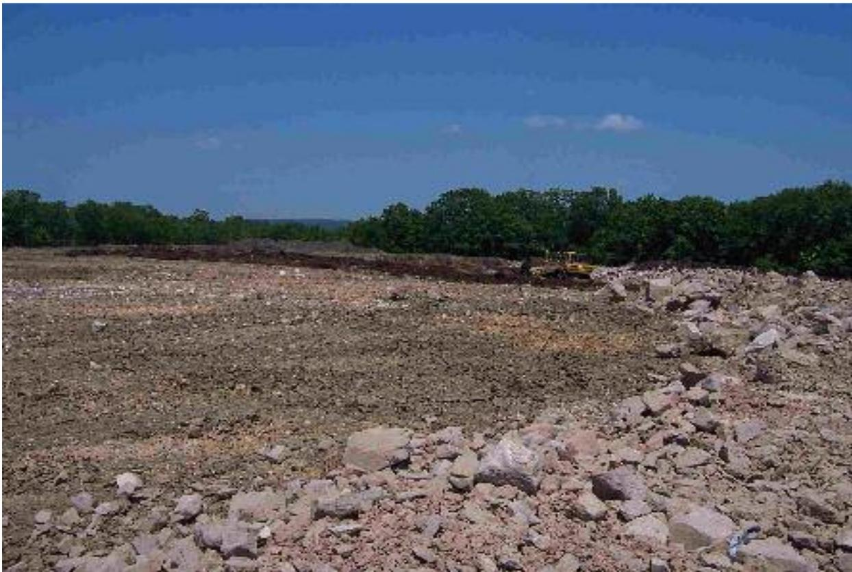
Figure 5-10. Preparation of Laydown Area 1. The fill material from the upper reservoir (sediment and concrete debris) was used to level the site. A hardfill cap will be placed over the top of the area. (Source: FERC Staff)
