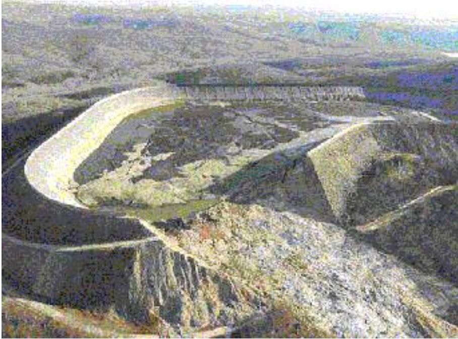
Figure 5-5. View of bedrock within, and immediately below failed embankment section. Note distribution of weathered rock (red-brown color) and topsoil (green-brown color). (Source: MDNR)
