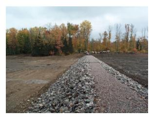
In the fall of 2002, Dike No. 2 was removed and a fuse plug was constructed in the general area. A fuse plug is an engineered earthen section that is designed to fail sacrificially in order to prevent a more catastrophic failure of the main dam. This action was taken because the project spillway did not have sufficient capacity to pass any more than 20 percent of the required design flood. The design
