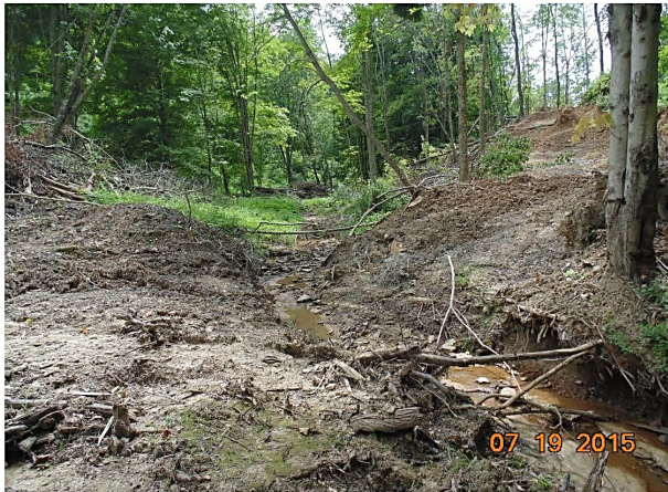
Stream crossing at Stonewall Gathering Pipeline construction site on Elk Lick Rd., 6.25 miles west of I-79 in northern Lewis County, WV
