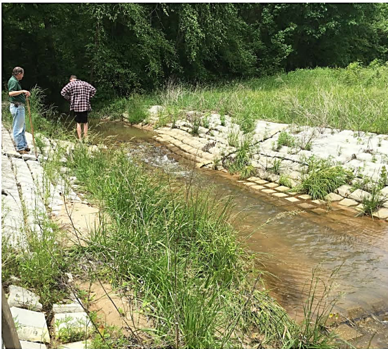
View of concrete mesh through creek in Pittsylvania County, VA
