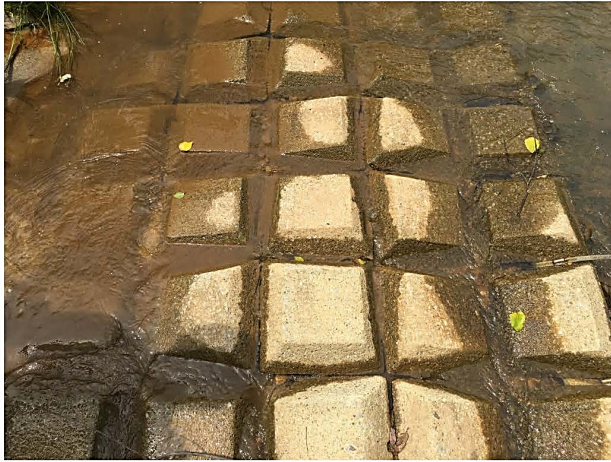
Concrete mesh covering exposed pipe along a pipeline ROW in a Pittsylvania County, VA creek
