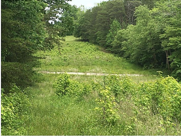
Easement ROW – white is the concrete mesh covering the pipes.
