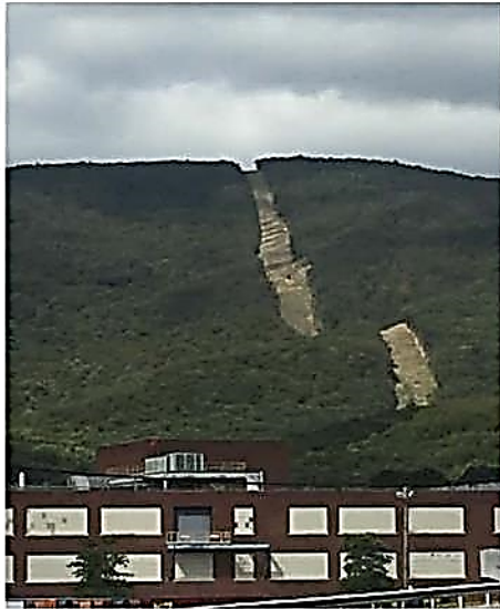
Figure 3. The deforested corridor caused by construction of the Columbia Gas pipeline in Giles County, Virginia. The photograph shows that the deforested corridor's width influences its visibility. In the foreground is the Celco plant, Giles County. (Photo by Brian Murphy, used by permission).
