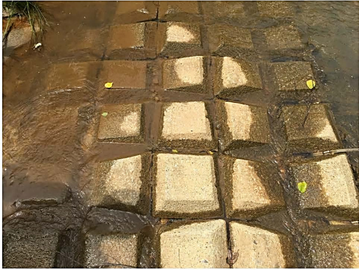
The concrete mesh – photo taken May 2016
