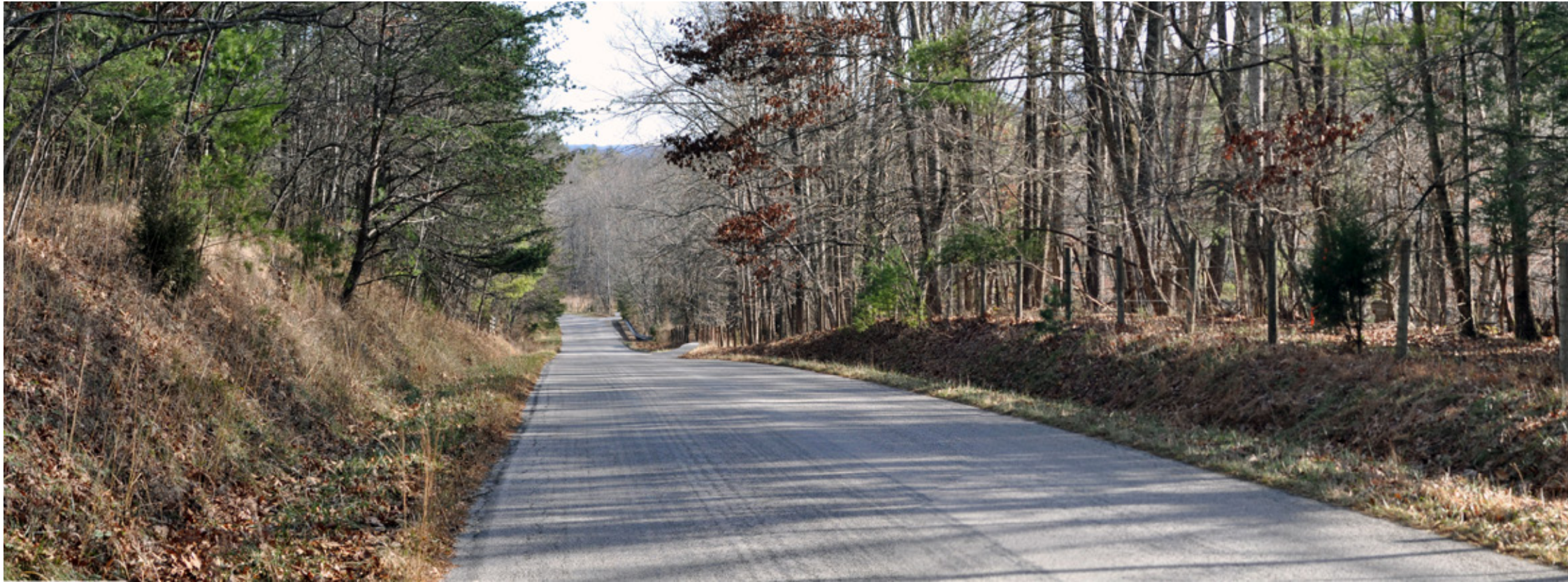
Post Construction (Leaf-off conditions) - The proposed pipeline would cross Craig Creek Road approximately 75 feet east of KOP PT-26. However, the pipeline would be bored under the road and the bore pits would be located approximately 60-100 feet from the road and would be screened by vegetation and terrain.
