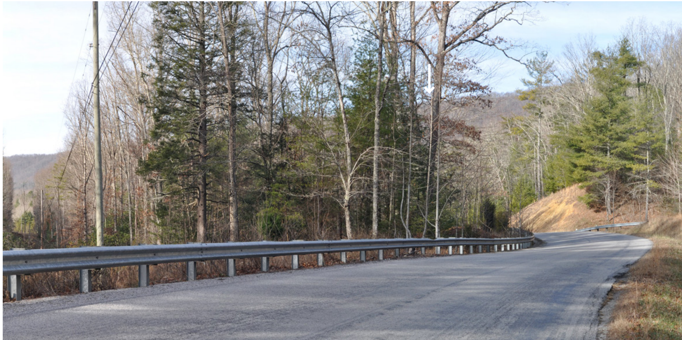
Post Construction (Leaf-off conditions) - The proposed pipeline crossing Brush Mountain and the adjacent valley would be screened by vegetation. The white arrow indicates the direction in which the proposed pipeline would cross over Sinking Creek Mountain approximately 0.8 mile from this viewpoint. Views would be screened by terrain and vegetation.
