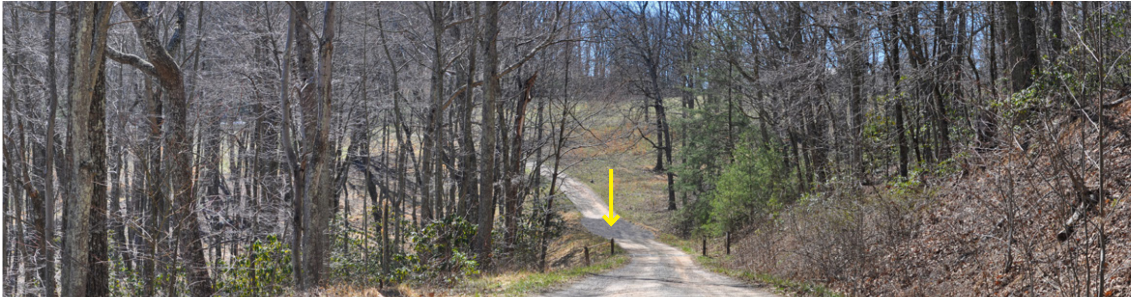
Post Construction (Leaf-off conditions) - From this location modifications to the roadway would be apparent where culvert upgrades would occur. The yellow arrow indicates the modifications to the roadway.
