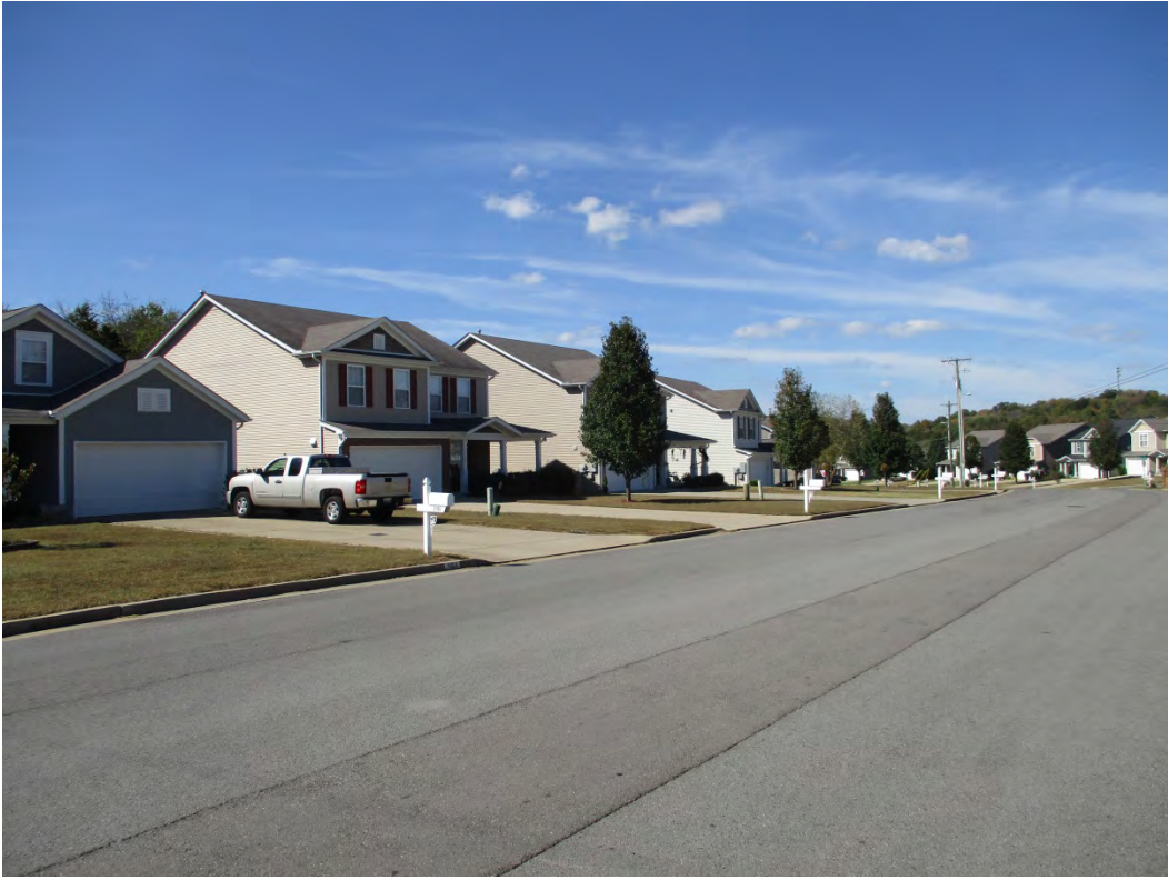
Figure 16. Hidden Creek Subdivision, Photo Point 26
