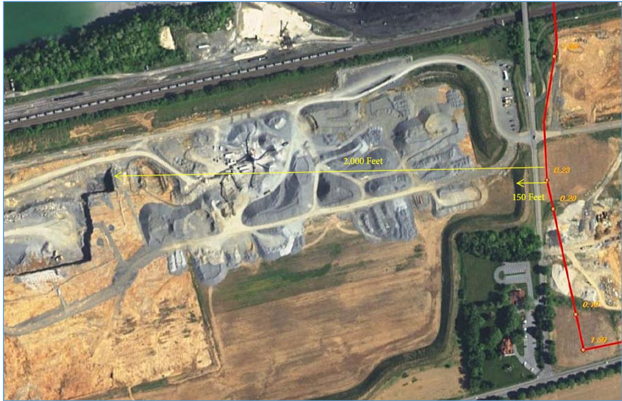
Figure 4.1.7-1 Stone Quarry With Material Storage and Handling Area Near CPL South Milepost M-0183 1.0
