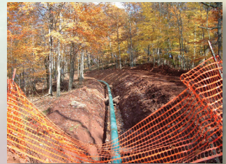
Pipeline in trench
