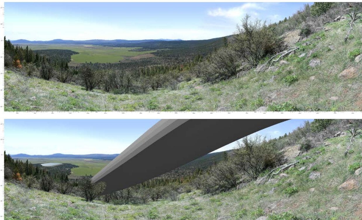
Figure 3-18. Photo-simulation of the penstock and lower reservoir as seen from KOP 26 (Source: Swan Lake North Hydro, 2015, Appendix E-18.24).
