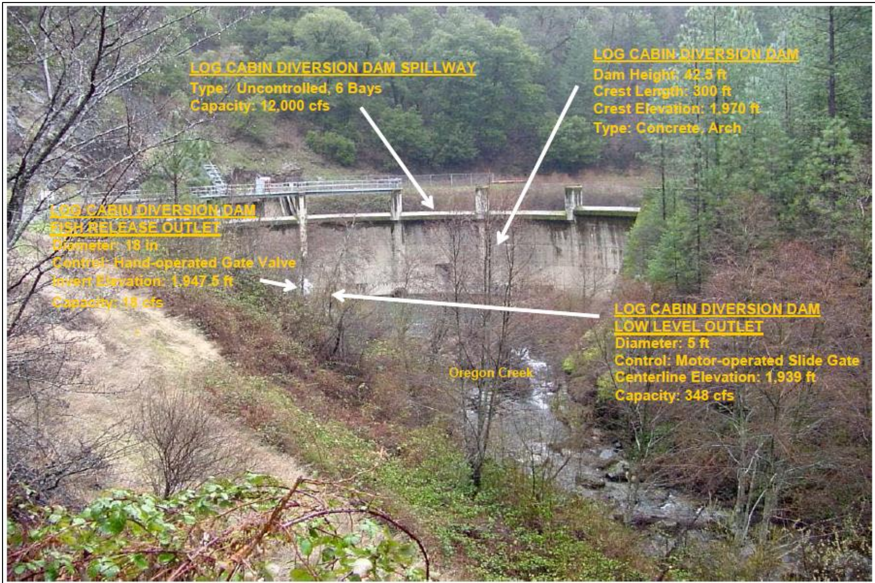
Figure 2-2. Log Cabin Diversion Dam (Source: YCWA, 2017a).
