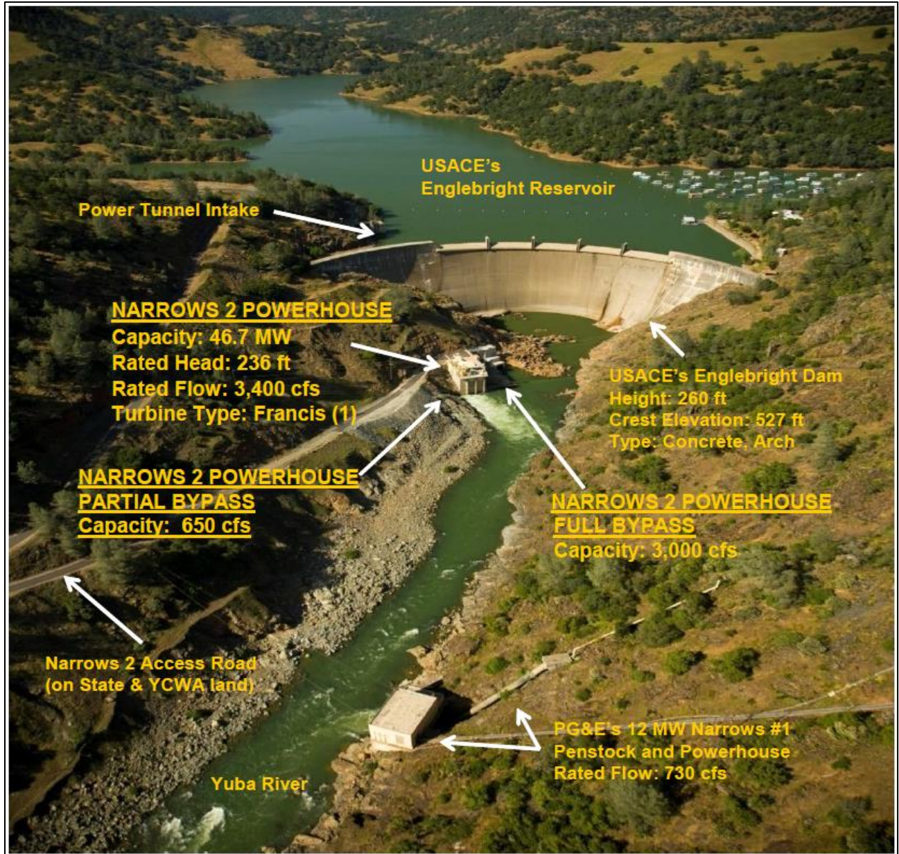
Figure 2-5. Narrows 2 Powerhouse, partial bypass, and full bypass and Englebright Reservoir and PG&E's Narrows 1 Powerhouse (Source: YCWA, 2017a).
