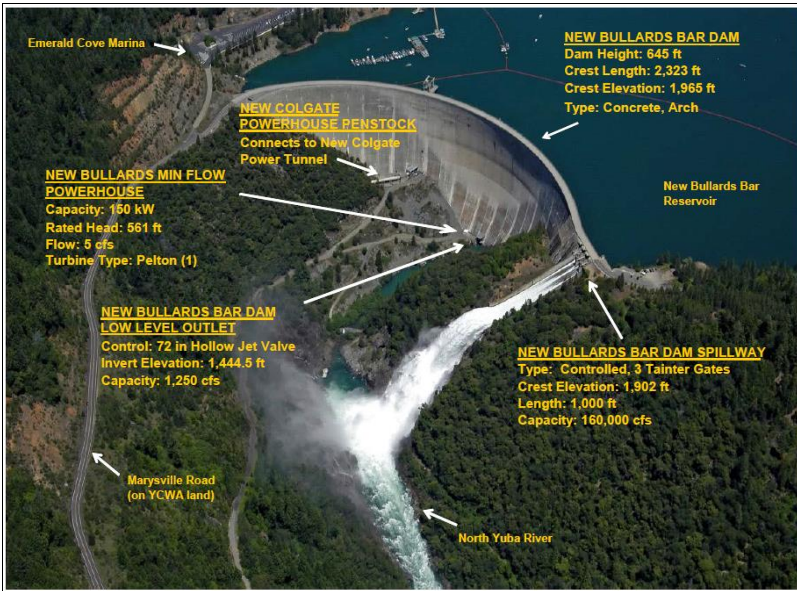
Figure 2-3. New Bullards Bar Dam and Minimum Flow Powerhouse (Source: YCWA, 2017a).
