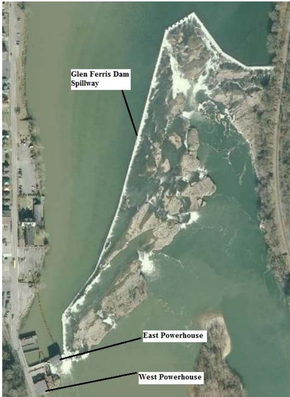
Figure 3. Glen Ferris Dam and Powerhouses (Source: license application, as modified by staff).
