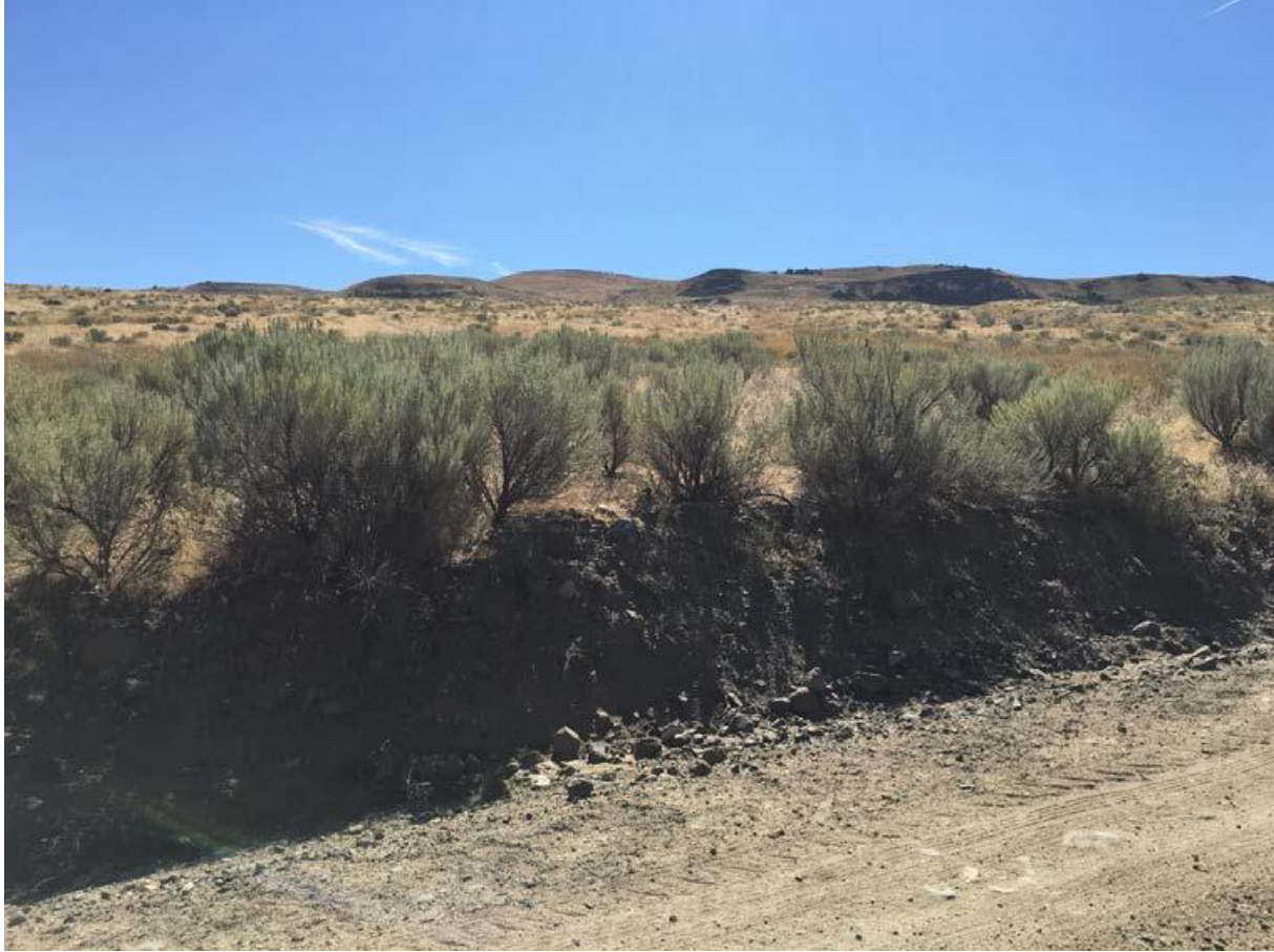
Figure 15. KOP 3 – view of location of penstock and upper reservoir tank site (source: application).
