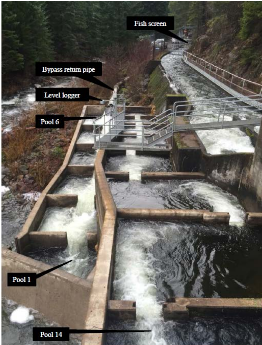
Figure 4. Photograph of the Prospect No. 3 Project diversion dam fish ladder and diversion canal, looking downstream from diversion dam during high flow conditions (Source: PacifiCorp, 2016c).
