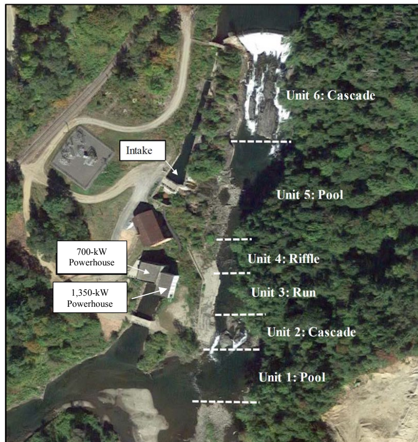
Figure 4. Great Falls Project bypassed reach mesohabitats. (Source: Lyndonville).
