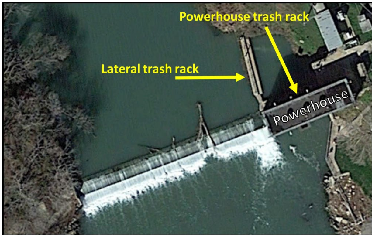
Figure 3-13. Location of project trash racks (Source: Google Earth, 2014; as modified by staff).
